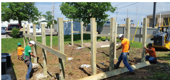
Workers preparing the frame for the new deck
